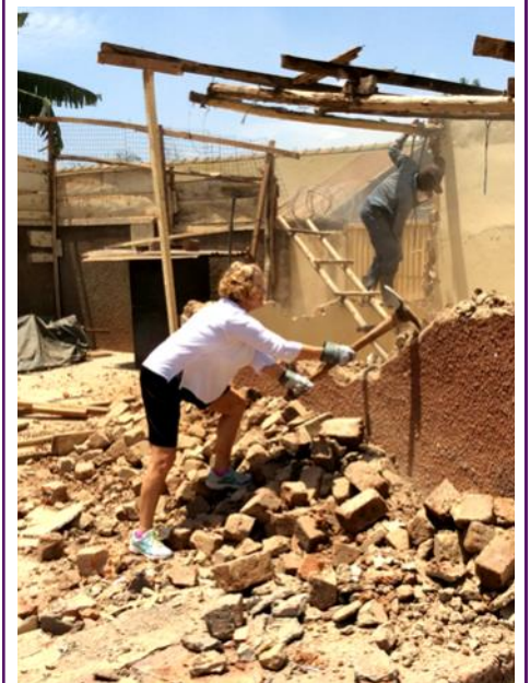
Betty helping to tear down old building.
