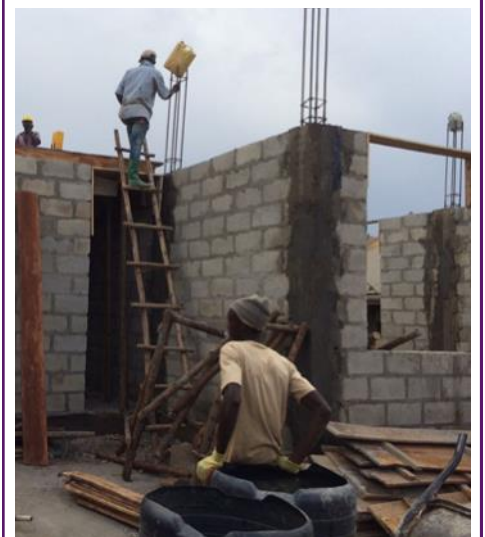
New building under construction.
