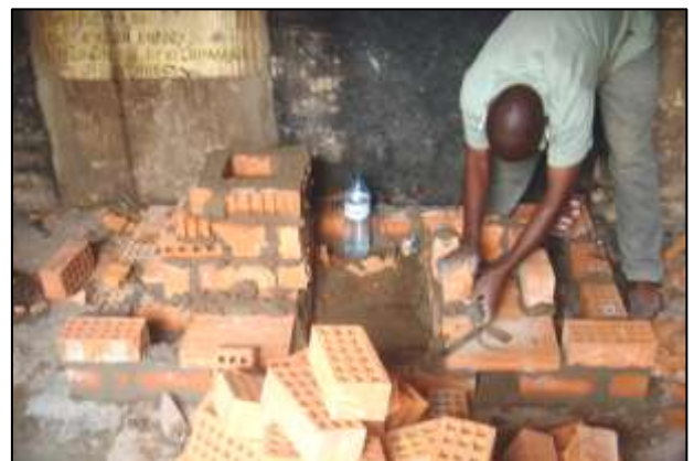
Patrick Bisere, Director of Prime Energy and Environment Savers Ltd., builds new institutional "Rocket" stoves for the school.
